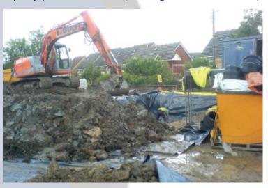
The soils were then backfilled into the pit as the groundworkers applied SpillAway Liquid Remediact and Dry Remediact directly to the soil.
